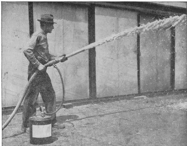
Fig. A-11-53. Air Foam Playpipe.
