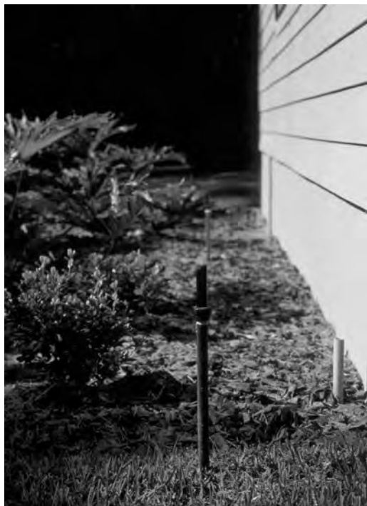
FIGURE A.24.3.4.1(b) Use of Low Volume Sprinklers in Organic Material. (Courtesy of Firewise Communities Program. Photo by G. Johnston.)
