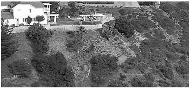
FIGURE A.25.1.3.3(a) Noncombustible Barrier on the Edge of a Downslope. (Courtesy of Firewise Communities Program. Photo by J. Smalley.)
