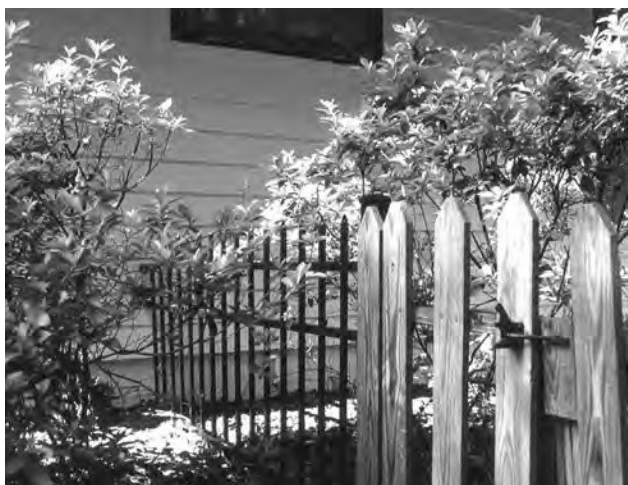
FIGURE A.24.3.4.3(b) Transition Fence Separates Combustible Fence from Structure. (Courtesy of Firewise Communities Program. Photo by G. Johnston.)
