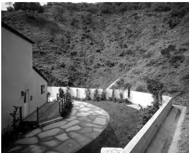
FIGURE A.25.1.3.3(b) Noncombustible Barrier Behind a House on the Edge of the Upslope. (Courtesy of Firewise Communities Program. Photo by J. Smalley.)
