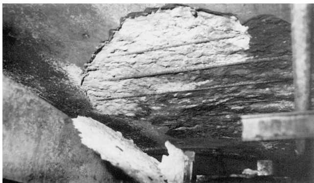
FIGURE 6.6.1.4 Spalling on Ceiling.
