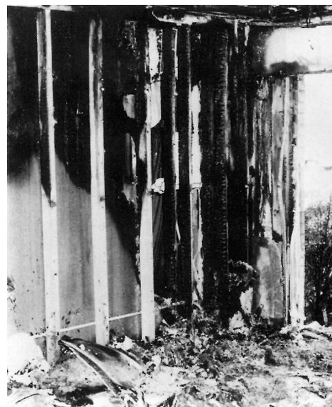
FIGURE 6.17.2 Typical V Pattern Showing Wall and Wood Stud Damage.
