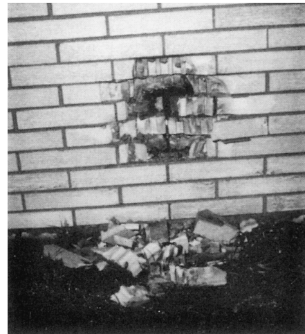
FIGURE 6.20.2 Damage to an Outside Brick Wall Caused by Thermal Expansion of an I-beam in the Basement.
