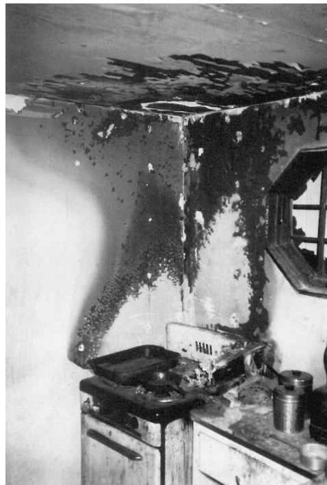
FIGURE 6.11 Clean Burn on Wall Surface.
