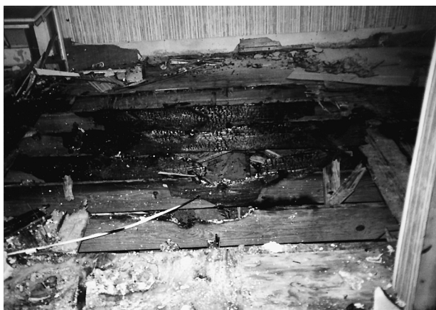
FIGURE 6.17.11 Saddle Burn in a Floor Joist.
