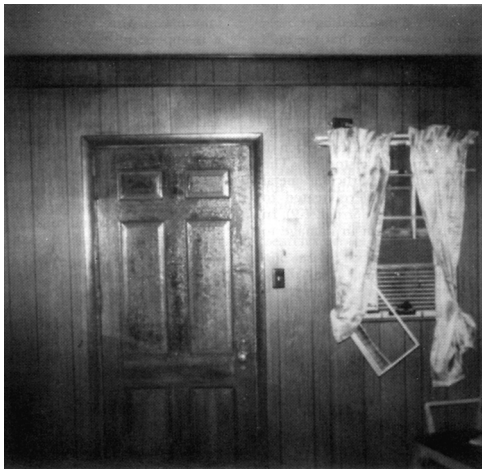
FIGURE 6.19.2.3 Blistering of Varnish on Door and Slight Scorching of Draperies, the Only Indications of the Natural Gas Flash Fire.
